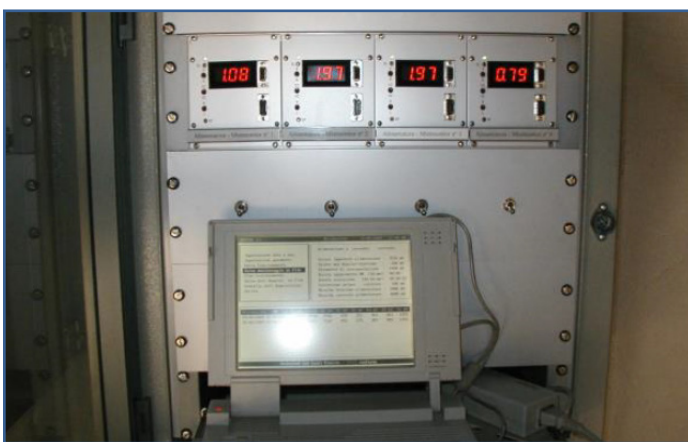
Feeding and Control Units for CP in concrete
