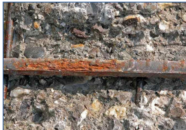
Fig. 2 - Example of corrosion attack on a rebar
