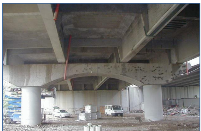
Bridge architraves protected by an ICCP system
