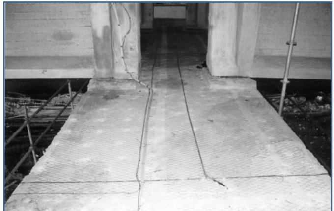
Ti-MMO mesh anode applied on a concrete pile
