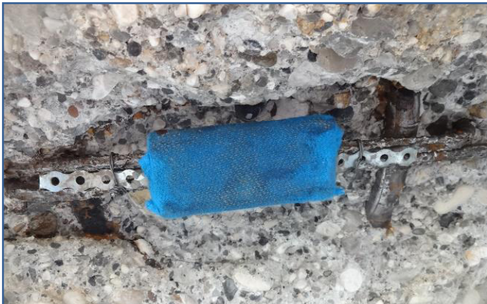
Zinc galvanic anodes for rebar cathodic protection
