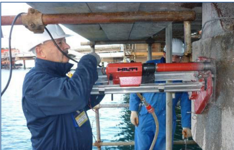
Fig. 5 - Core drilling
