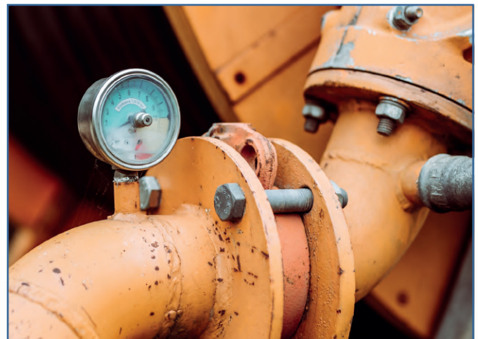
Fig.3 – Process controls and gauges are fundamental for IOWs purposes.
